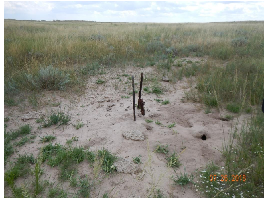
Photo 6: Photo taken from the access road, west of the location (GPS coordinates 39.77372/-102.88281). Photo shows pipe riser equipment remaining. Riser needs to be removed in accordance to 1004.a
