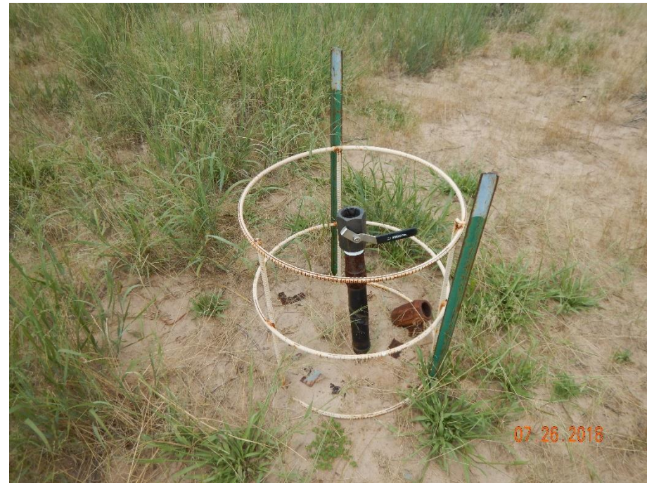
Photo 4: Photo taken from the west end of the location. Photo shows pipe riser remaining on location. Riser needs to be removed in accordance to 1004.a
