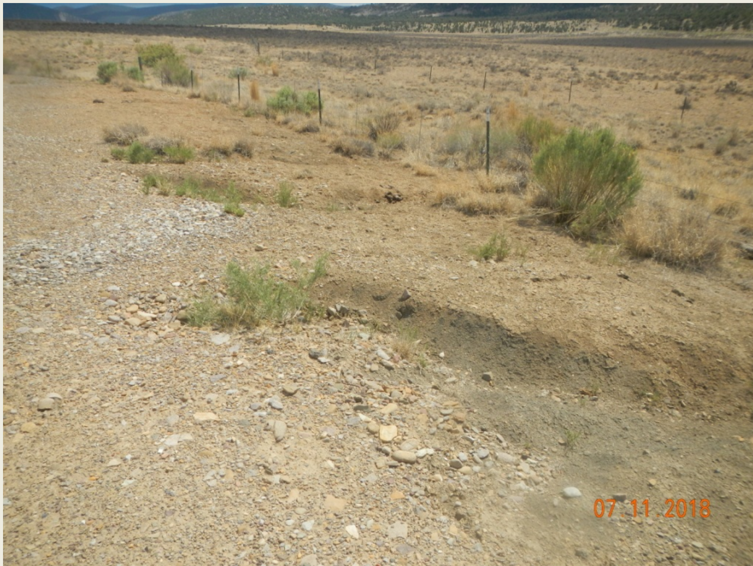
Photo 3. View of erosional channels forming within the southern project area. This needs to be monitored and stormwater controls installed if erosion worsens.
