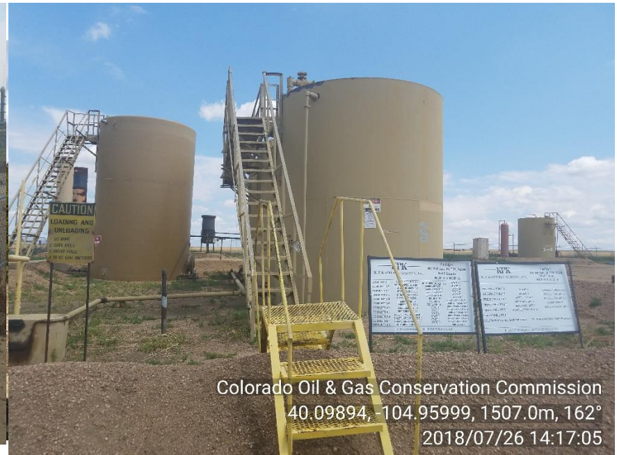
Photo 2. Tank battery
