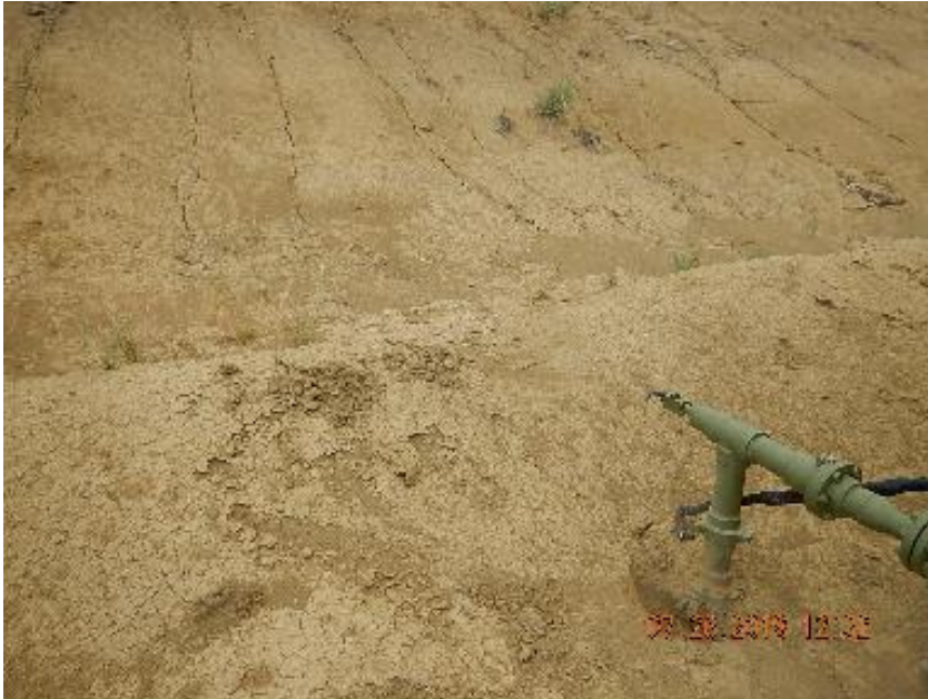
Photo 3: Breach in ditch and berm on cut slope.
