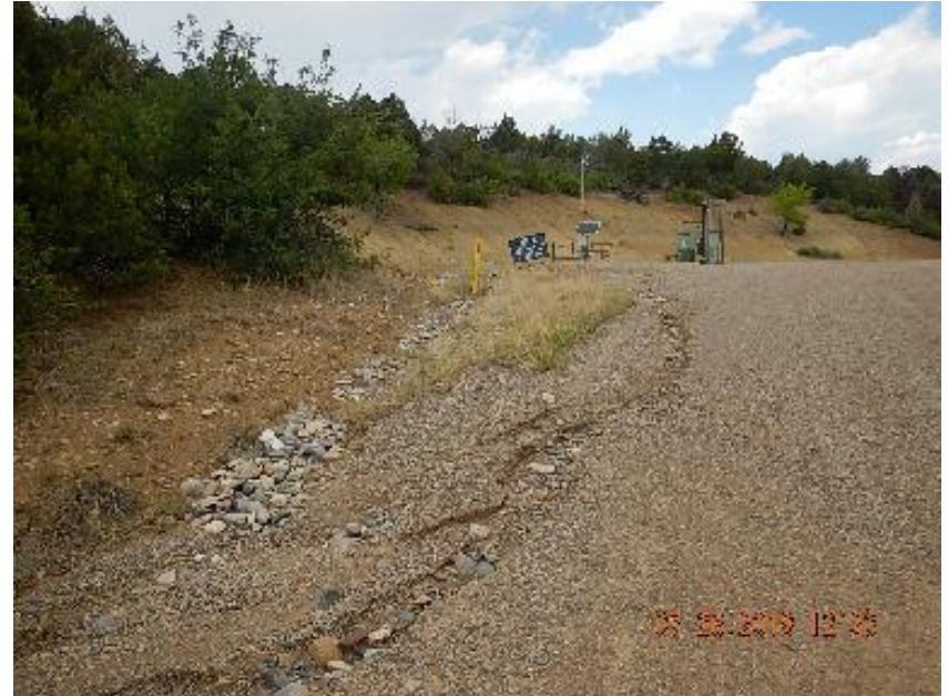
Photo 4: Erosion channel in access road at entry point.
