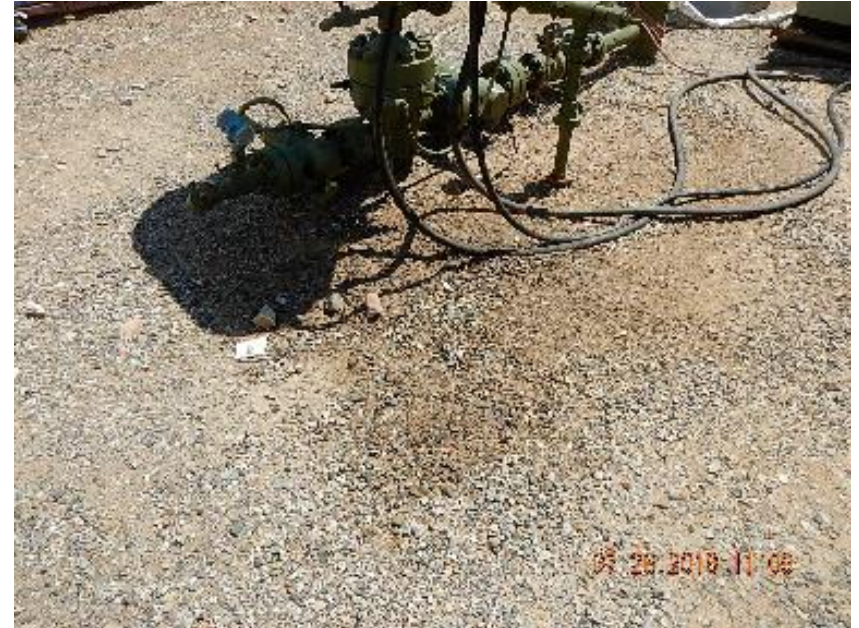
Photo 2: Impacted soil and gravel at wellhead.
