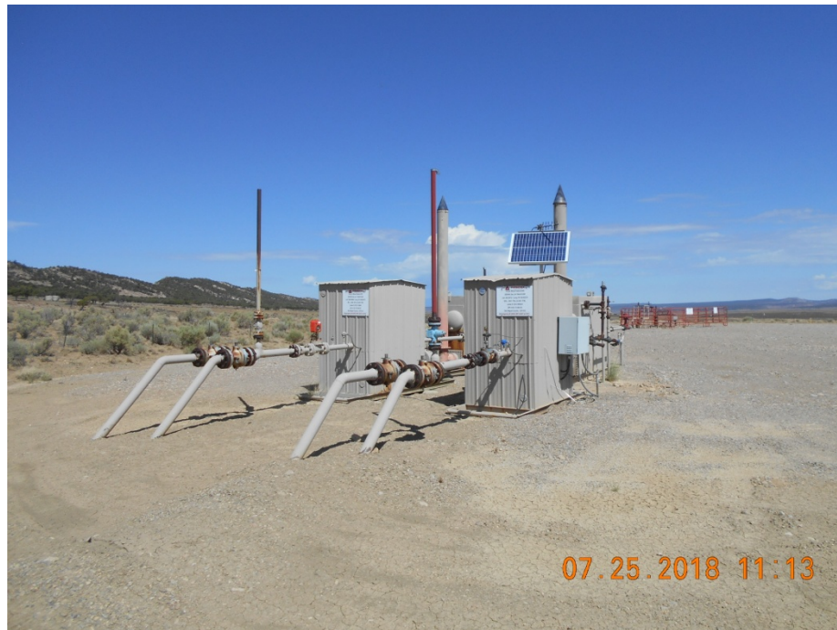
Separators and meter housings
