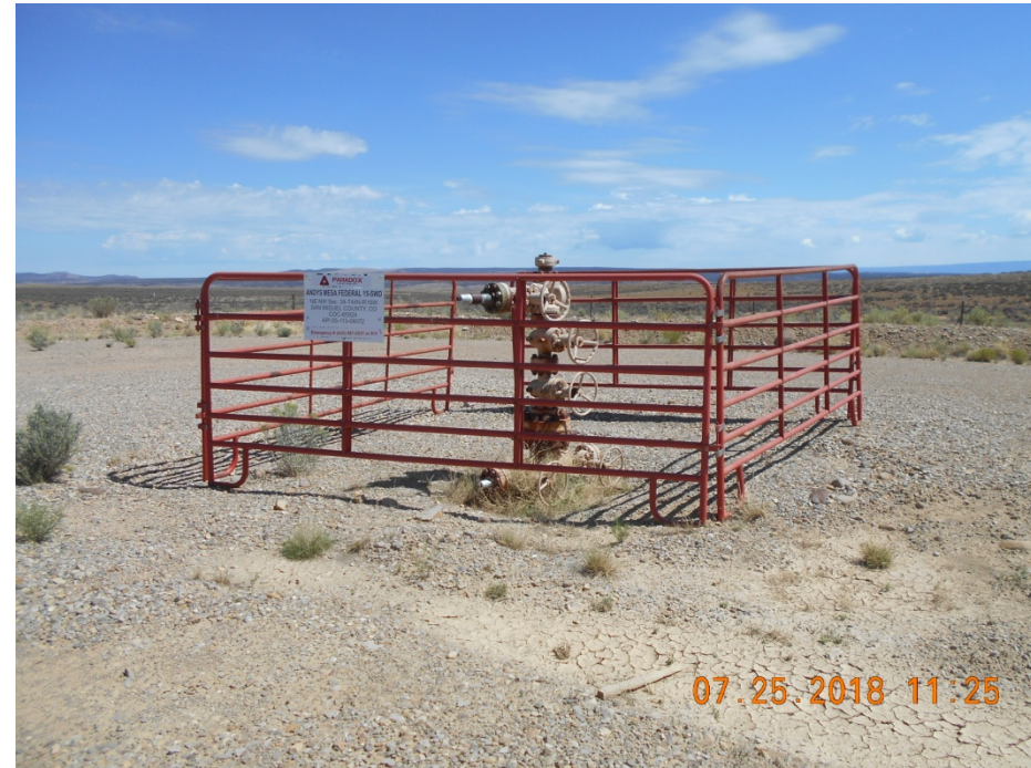
Injection Wellhead
