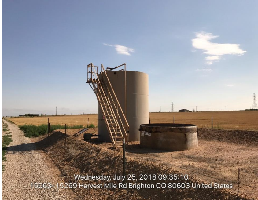
Photo#1 Production tank and produced water tank
