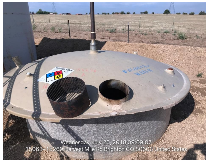
Photo#2 Corrective Action/Lid not on produced water tank
