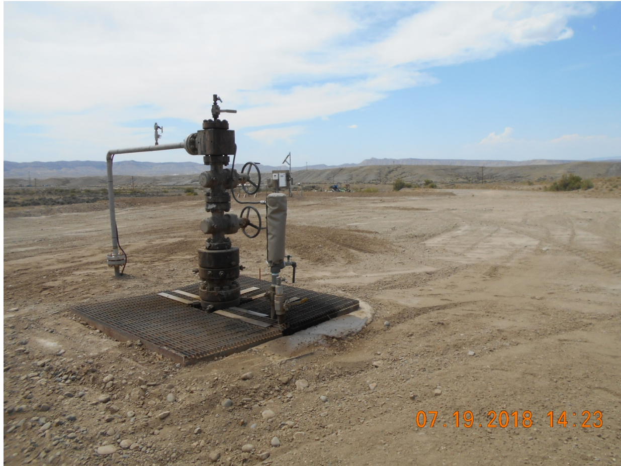
Injection Wellhead
