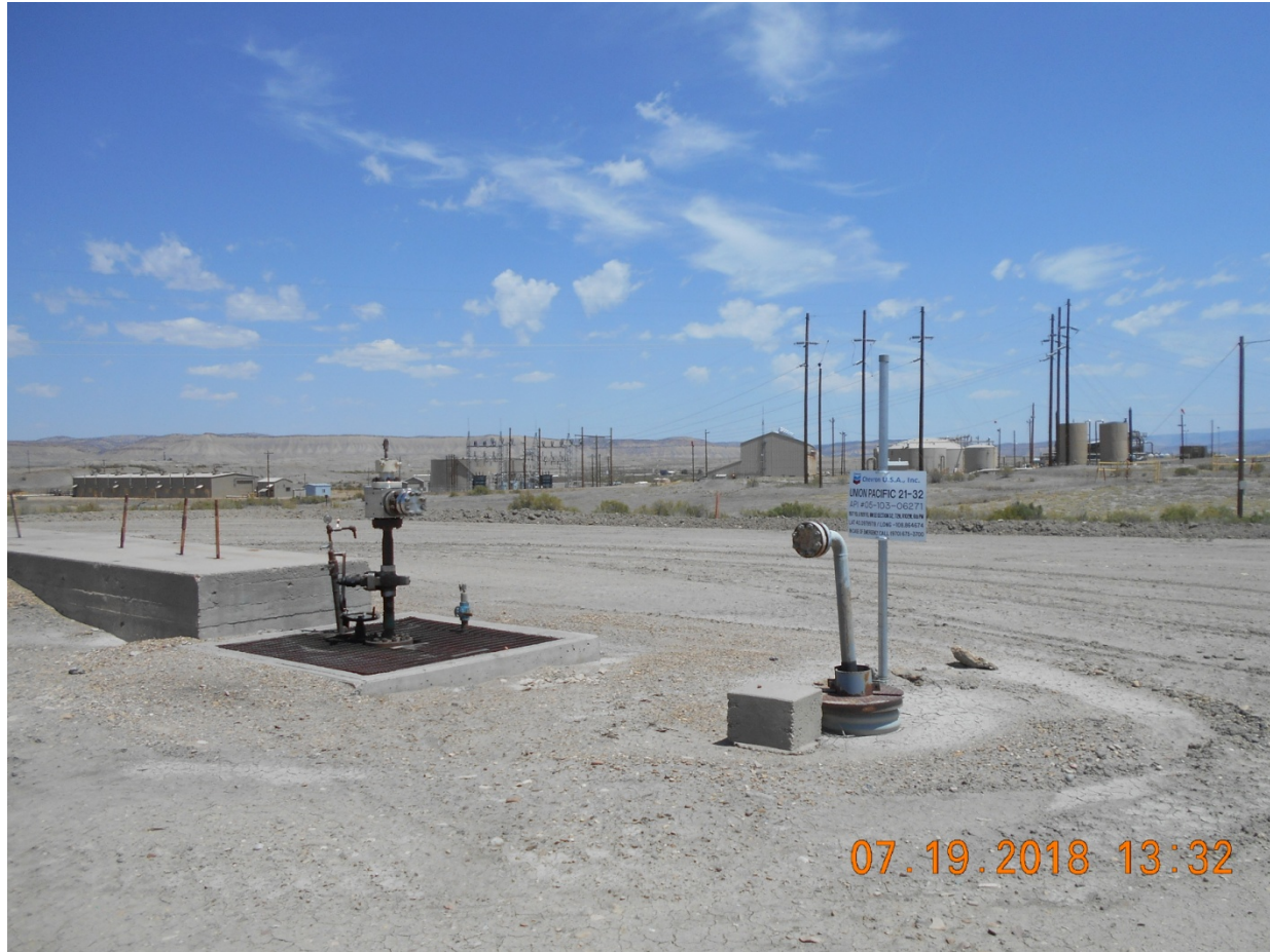
Injection Wellhead
