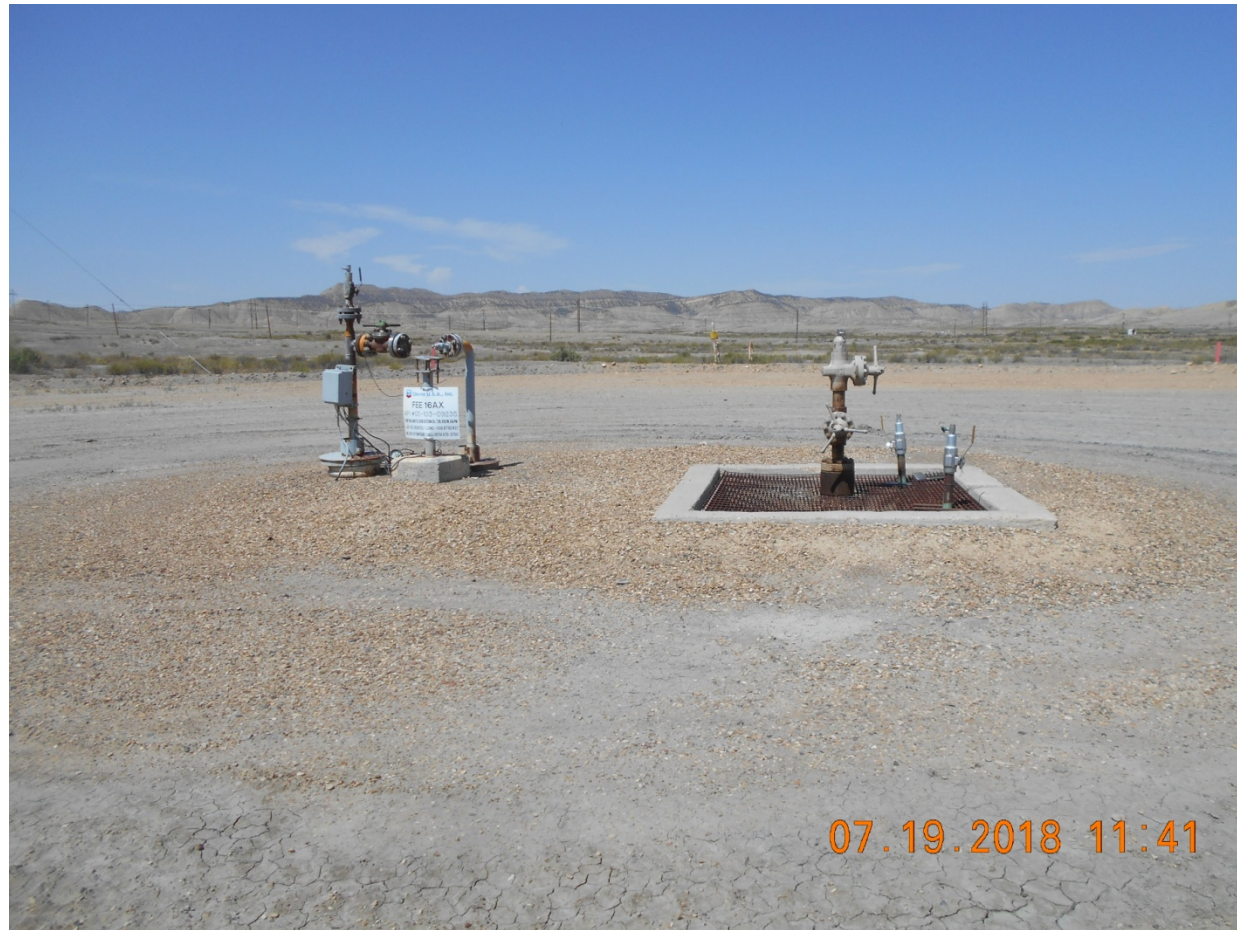
Injection Wellhead
