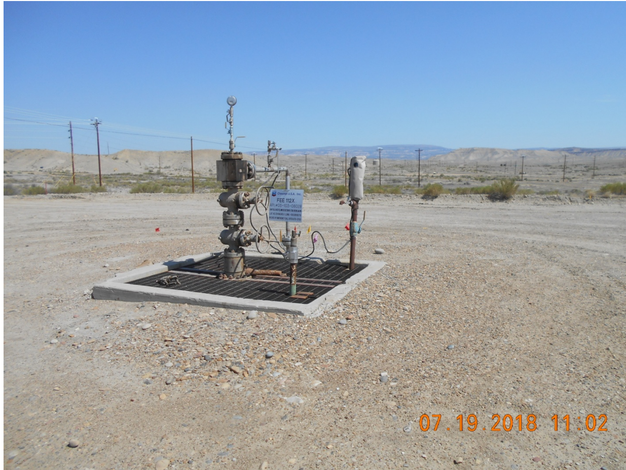
Injection Wellhead
