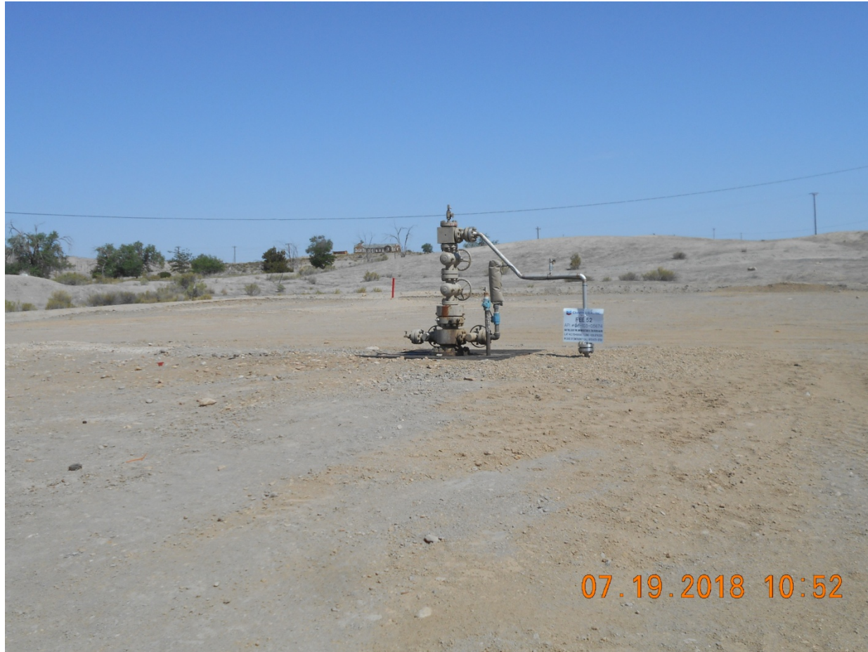
Injection Wellhead
