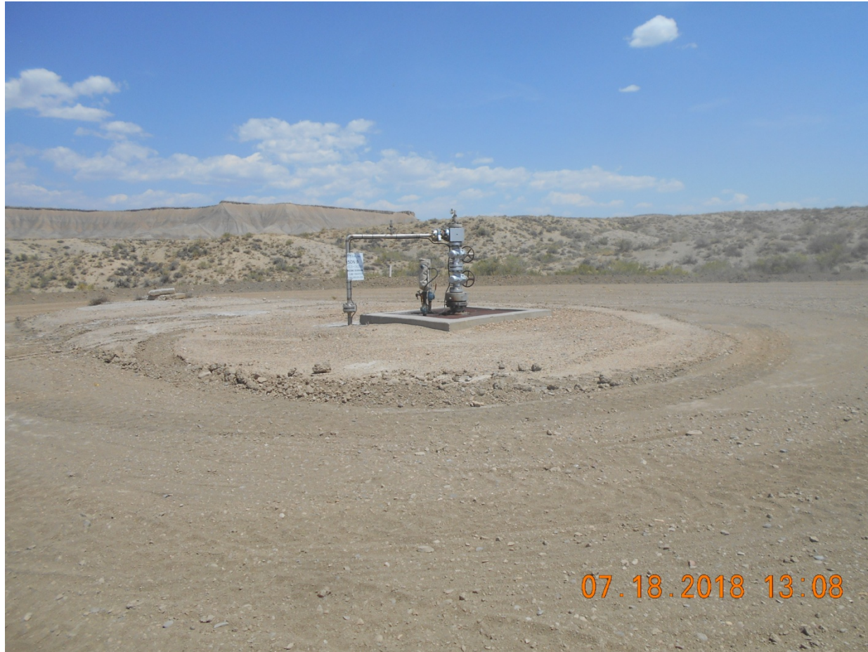
Injection Wellhead
