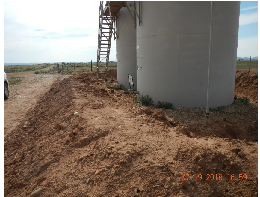
Secondary containment berm has been repaired.
