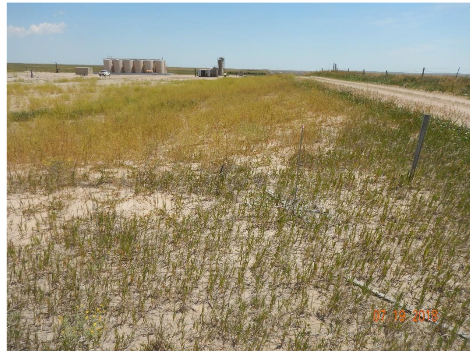
Photo 16: Photo taken from the topsoil berm on the southwest corner of the location, facing east. Photo shows areas on the west end of the location that do not appear to be necessary for production operations. These areas need to be reclaimed in accordance to COGCC 1003 interim reclamation requirements.
