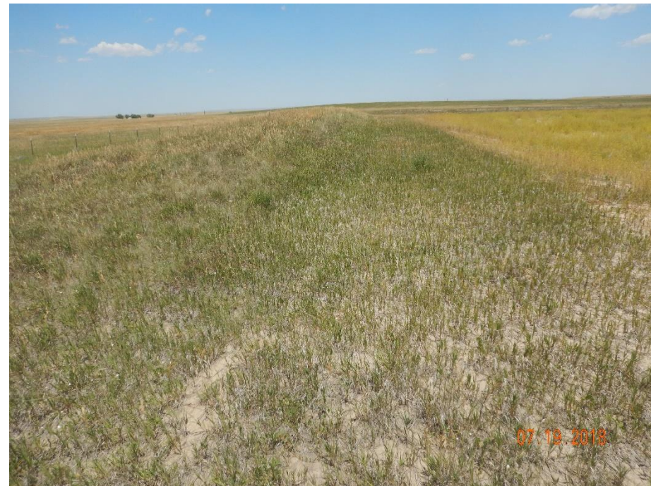
Photo 14: Photo taken from the topsoil berm on the southwest corner of the location, facing north. Photo of topsoil berm. Photo also shows areas on the west end of the location that do not appear to be necessary for production operations.
