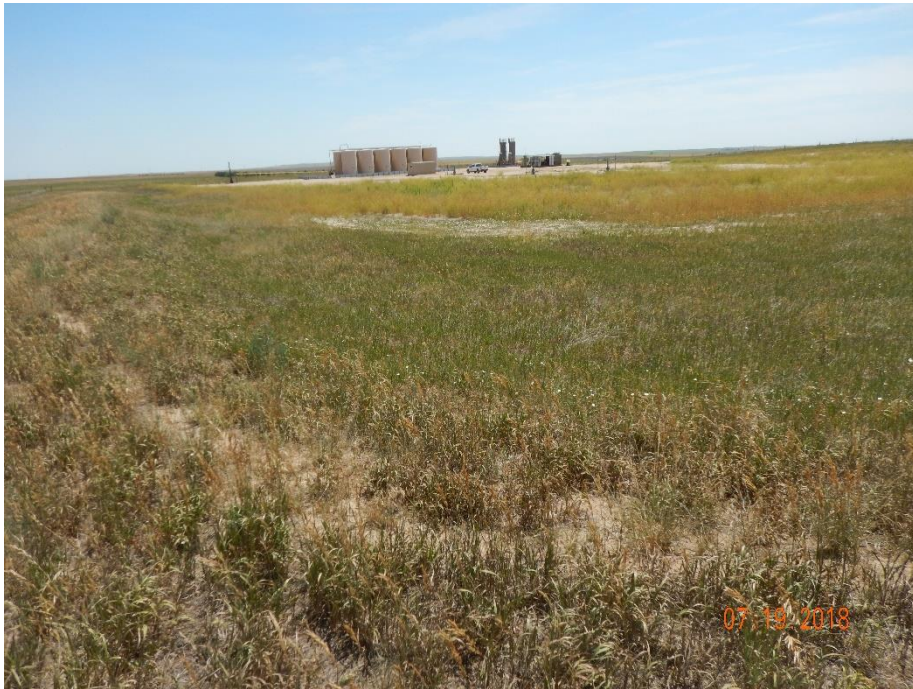
Photo 13: Photo taken from the topsoil berm on the northwest corner of the location, facing southeast. Photo shows areas on the west end of the location that do not appear to be necessary for production operations. These areas need to be reclaimed in accordance to COGCC 1003 interim reclamation requirements.
