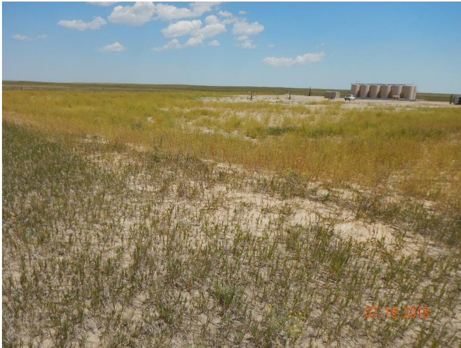
Photo 15: Photo taken from the topsoil berm on the southwest corner of the location, facing northeast. Photo shows areas on the west end of the location that do not appear to be necessary for production operations. These areas need to be reclaimed in accordance to COGCC 1003 interim reclamation requirements.
