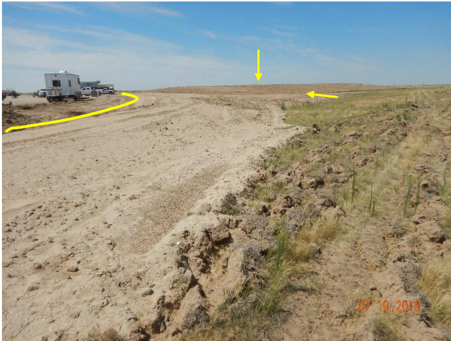
Photo 17: Photo taken from the north end of the locaiton, facing southwest photo shows perimeter stormwater ditch, soil stockpile and wattle BMPs. See comments under photo 13.
