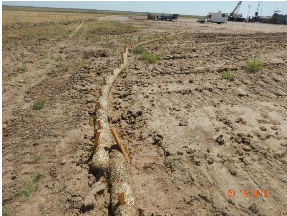
Photo 13: Photo taken from the north end of the topsoil stockpile. Photo shows straw wattle stormwater and sediment control along perimeter of the berm. Note that control has not been installed in accordance to good engineering practices; Wattles are required to be trenched and backfilled to be in proper functioning condition. Also note, the perimeter ditch runs partially on the southeast end of the berm, then travels to the northeast. Wattles appear to be the only control on the eastern/northeastern area of the stockpile. Unless appropriate measures are taken to ensure wattles are in proper functioning condition, the eastern/northeastern areas of the soil stockpile are at risk to sediment runoff and degradation.
