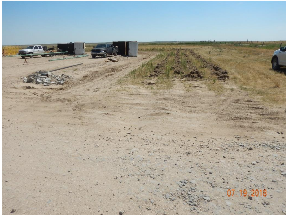
Photo 7: Photo taken from the south end of the location, facing east. Photo shows surface roughening used in conjunction with ditch along the perimeter of the location.
