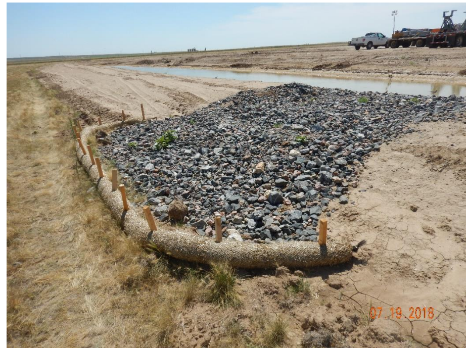
Photo 18: Photo taken from the south end of the sediment pond, facing east. Photo shows outlet appears to have sufficient outlet protections/armoring.
