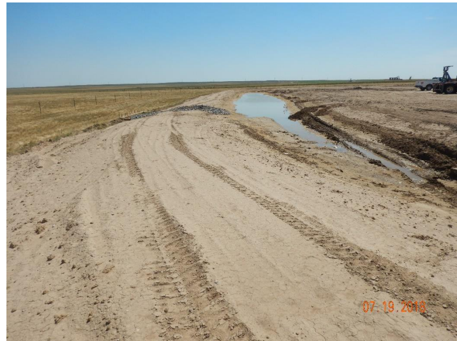
Photo 16: Photo taken from the North end of the location, facing south. Photo of sediment pond connected to the perimeter stormwater ditch.
