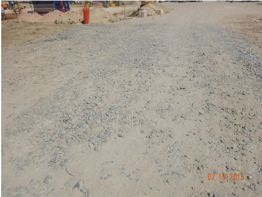
Photo 5: Photo taken from the access road. Photo shows tracking pad.
