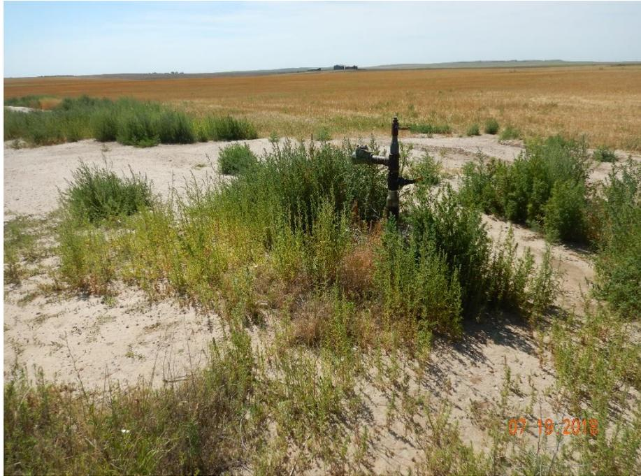
**Photo 1:** Photo taken from the battery location, facing southeast. Photo shows riser remaining on location. Riser is required to be removed in accordance to 1004.a
