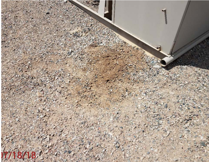
Location Photo #5, Stained ground by front of the vessel, south side.
