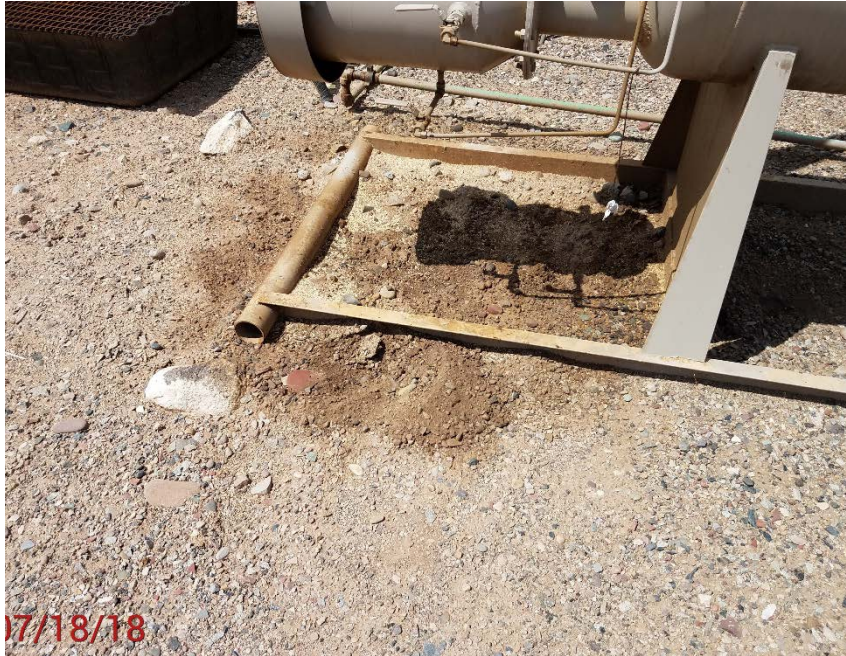
Location Photo #3, Stained ground under low stage vessel
