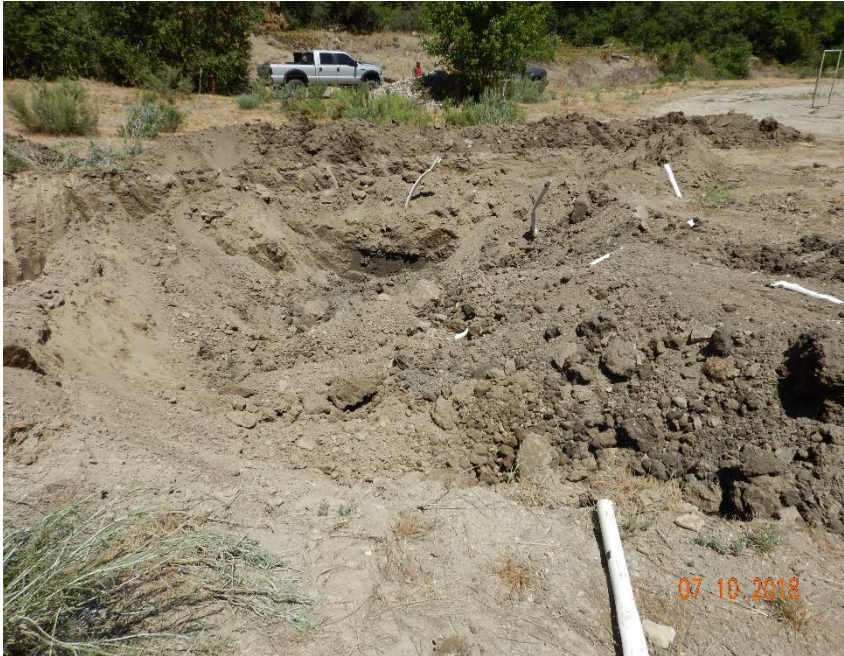
Photo #5 – View across excavation from SE with visibly-impacted soil.
