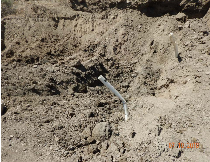
Photo #3 – PVC risers inside of excavation related to remediation attempt under previous operator using passive SVE system.
