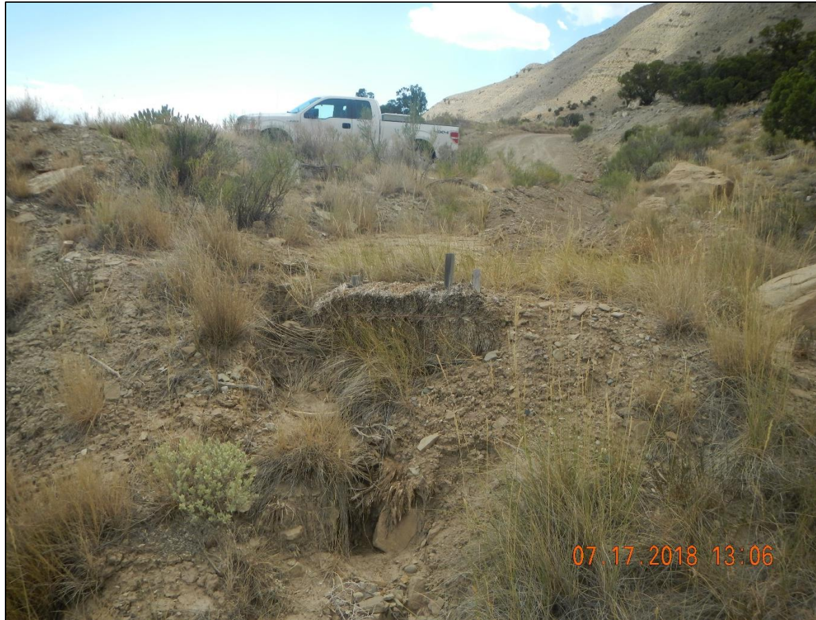
Sediment build up over straw bales used for check dams @ Switch back (39.48597 108.04075)
