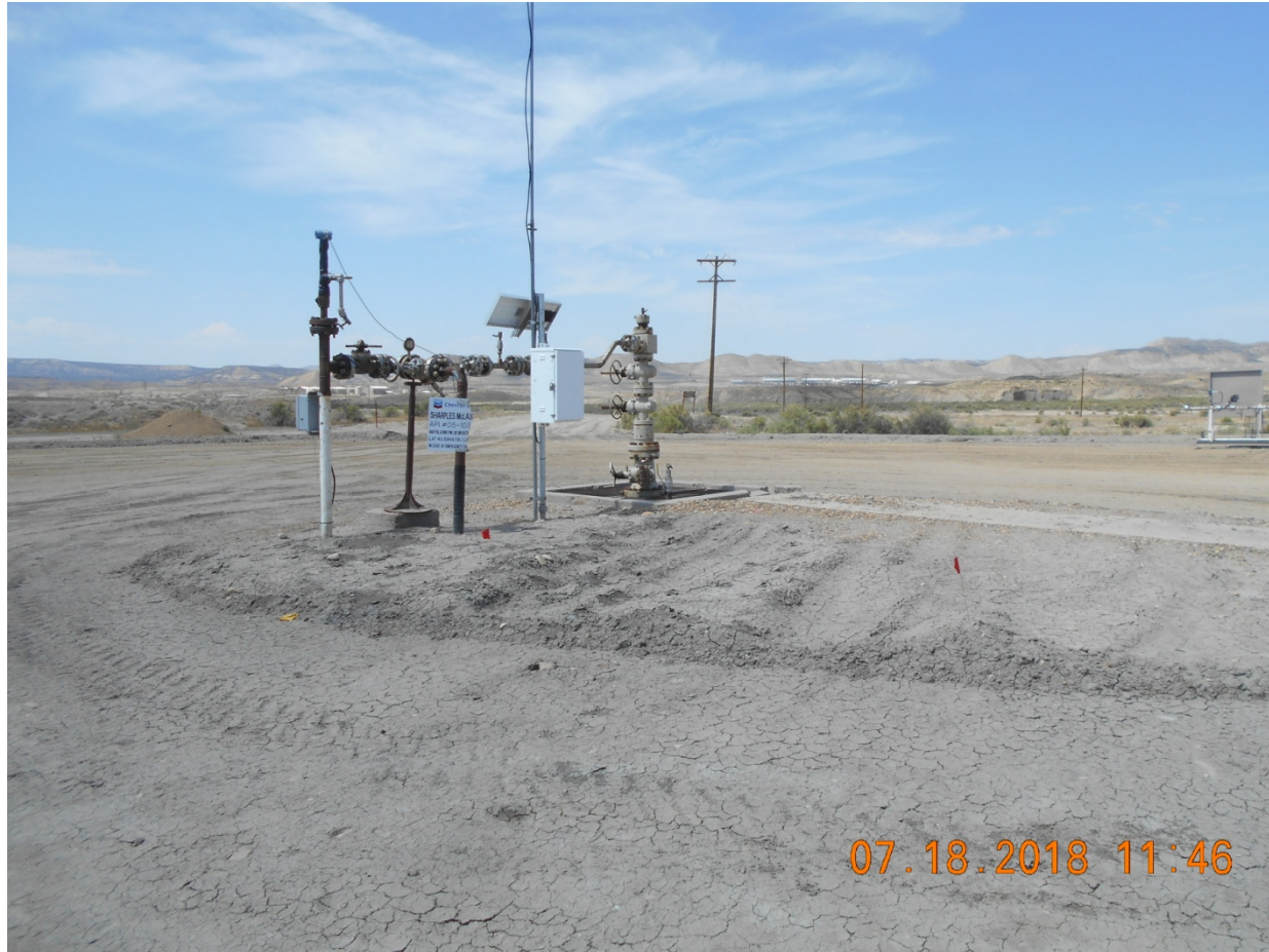
Injection Wellhead
