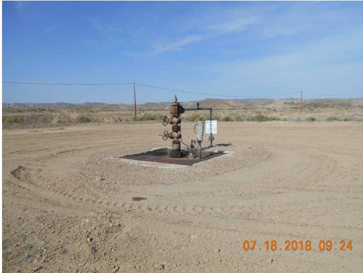
Injection Wellhead
