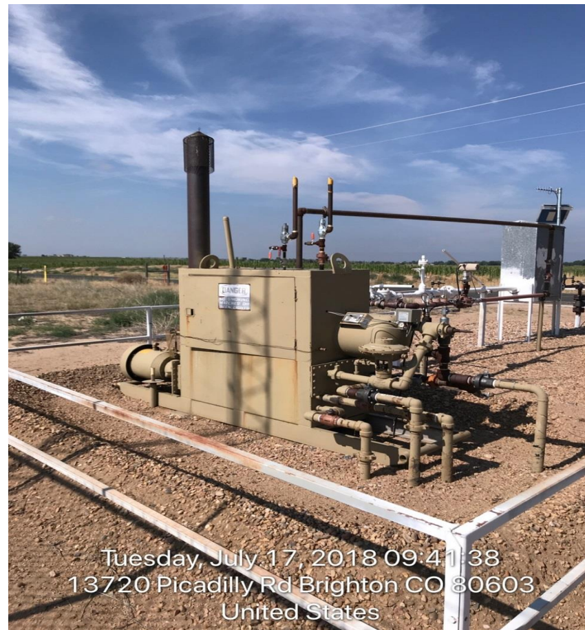
Photo#2 Separator/Meter/Automation RTU
