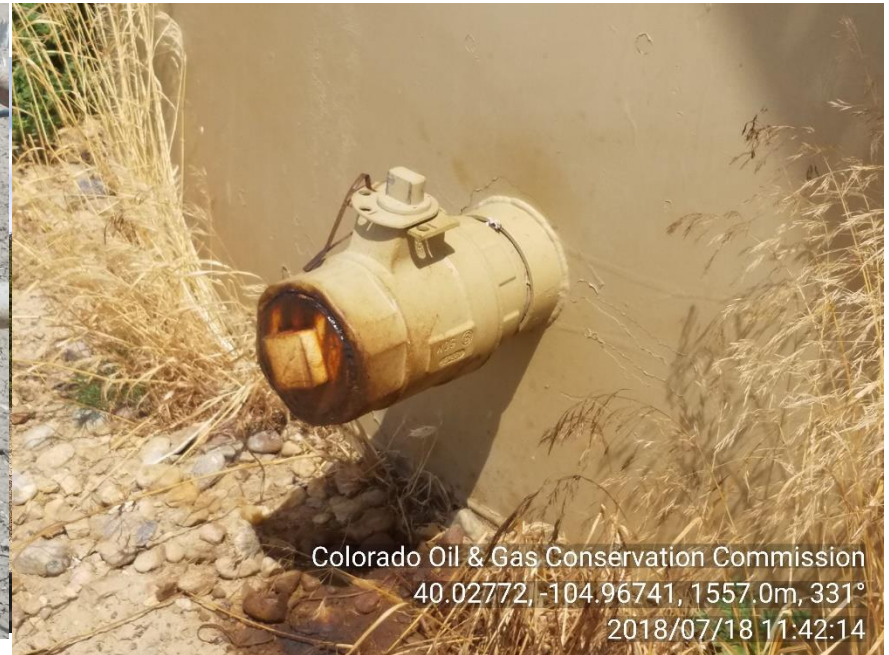
Photo 6. Stained soil under plugged 4" valve on crude oil tank
