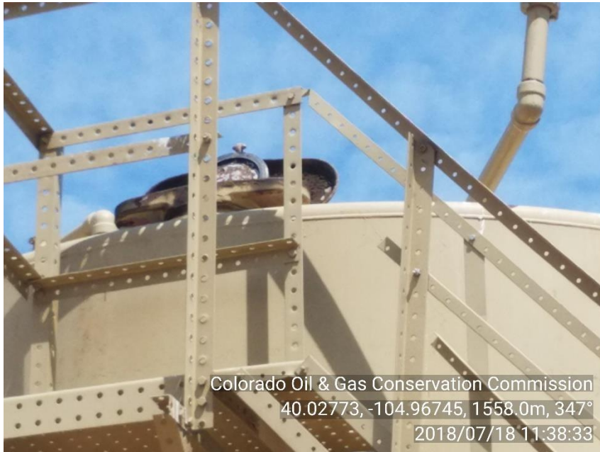
Photo 3. Vent hatch open
