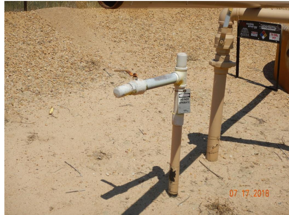
Photo 2: Photo taken from the northwest end of the tanks. Photo shows riser remaining.
