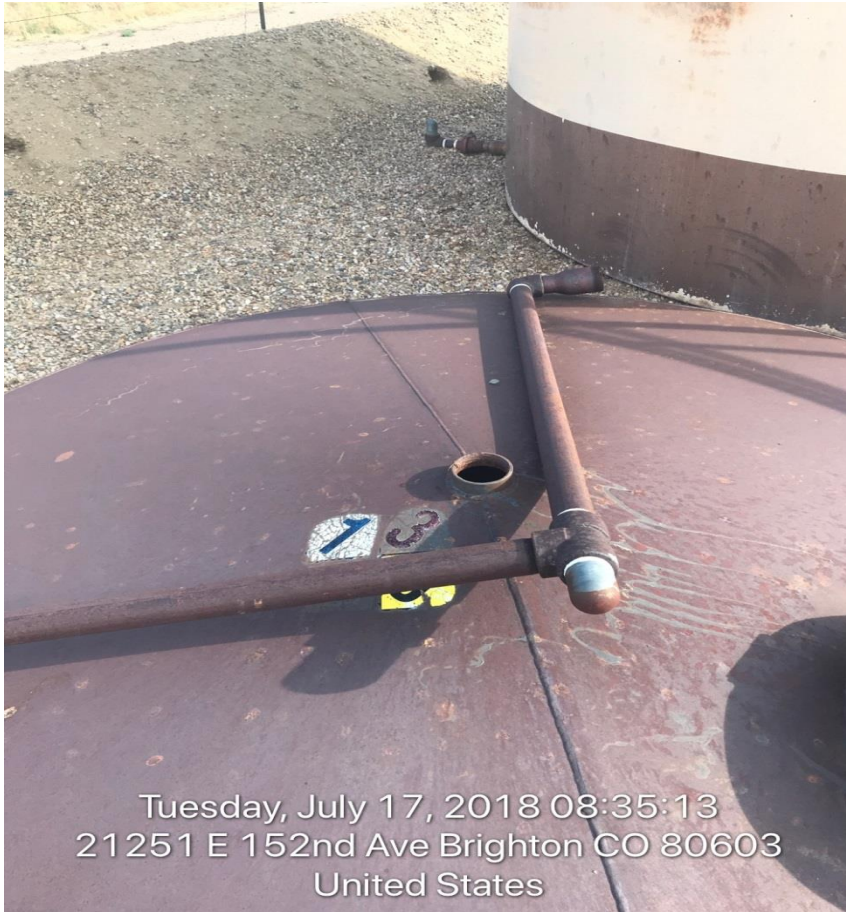
Photo#3 Pit with vent disconnected needs reinstalled or capped
