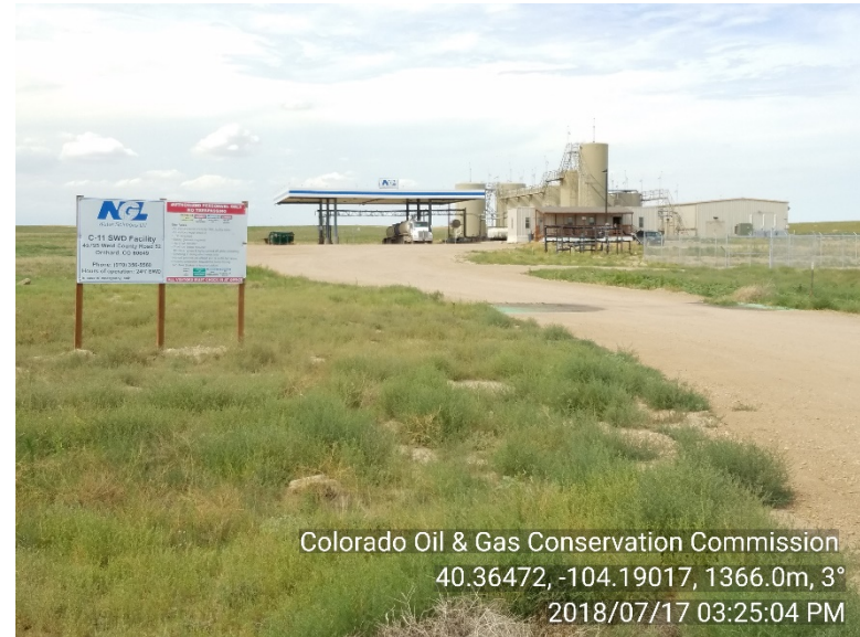
Photo #6 NGL C11 (API 05-123-38533) Injection Facility View 1
