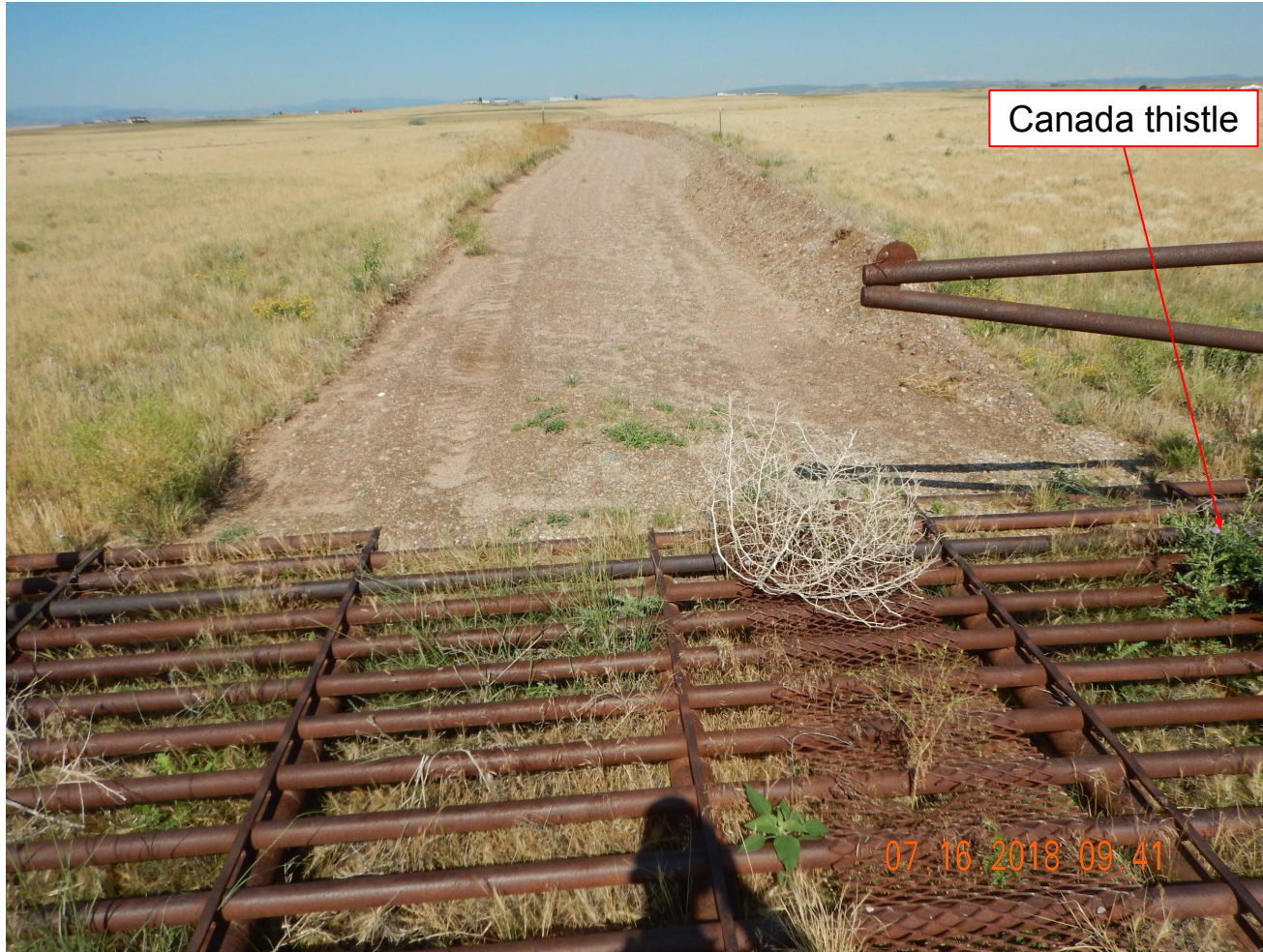
Photo 2. Photo taken from the entrance of the location off CR7, facing West. Final reclamation activities have not been performed on the access road. Appears gravel was scrapped off to the side of the access road but has not been removed, contoured or seeded. Operator shall perform final reclamation activities throughout the entire access road per Rule 1004. Canada thistle, a List B Colorado noxious weed, was observed at the entrance off CR7 and the well location entrance.
