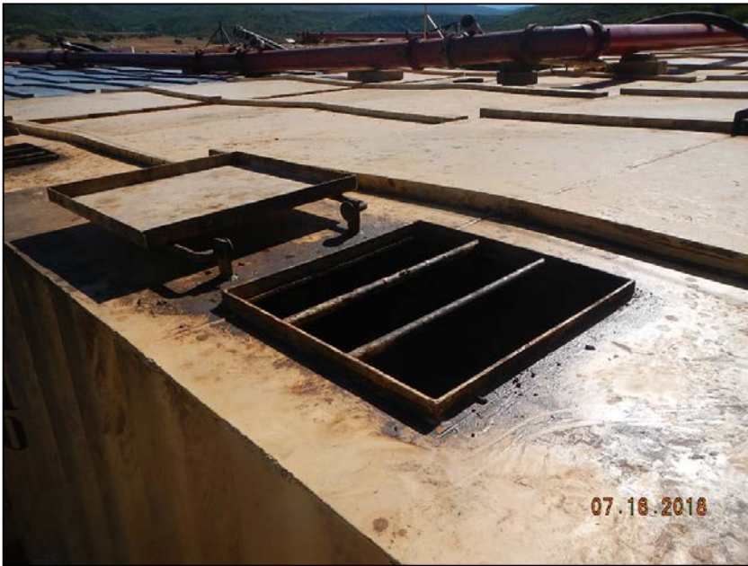
Photo 1. Open hatches on frac tanks.
