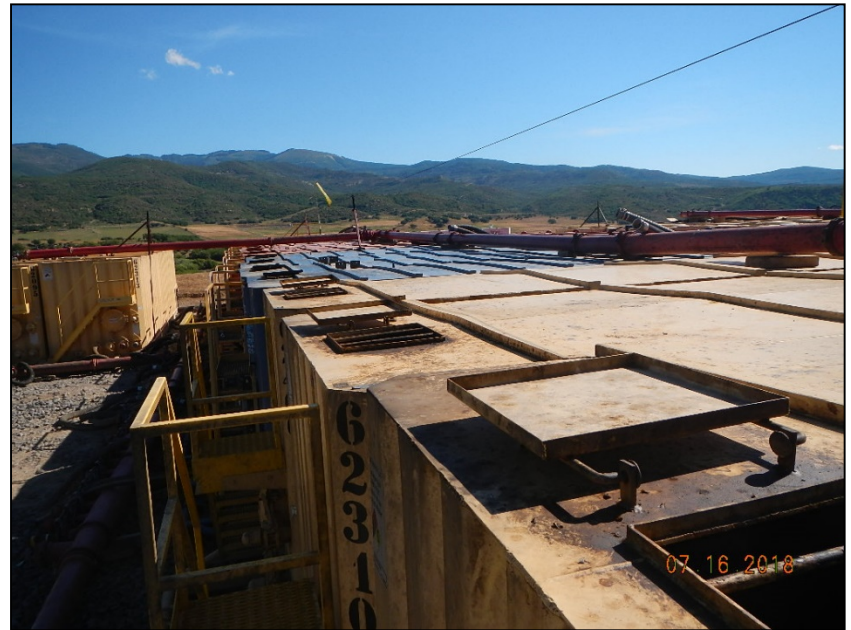
Photo 2. Open hatches on frac tanks.
