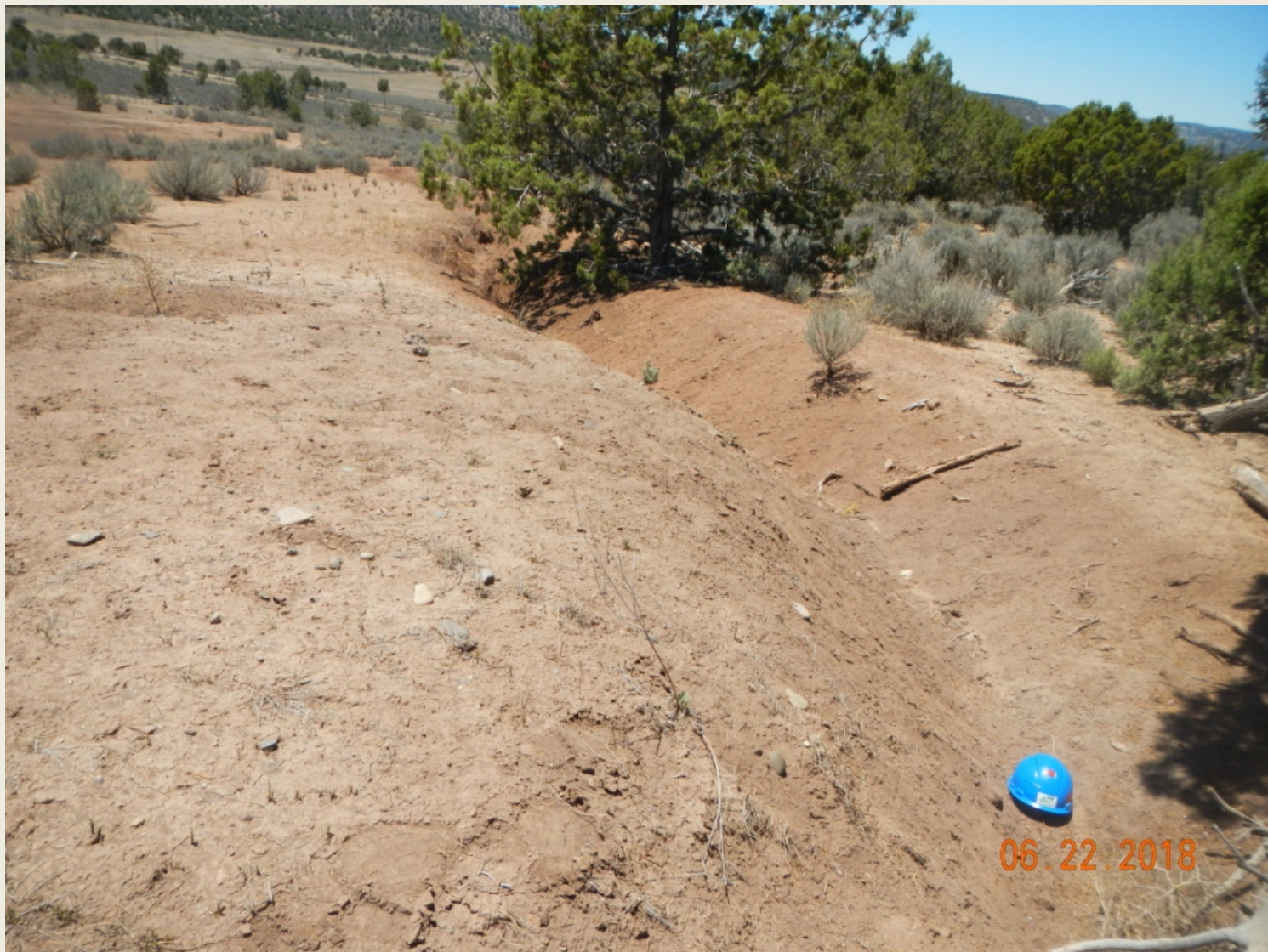
Photo 5. View of diversion in the northwestern project area needing stormwater controls to de-energize stormwater flows exiting the project area.
