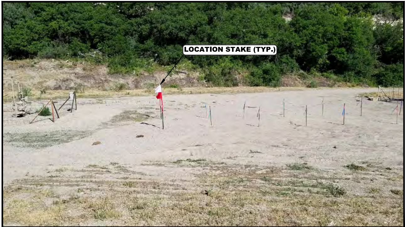
PHOTO: VIEW OF LOCATION STAKES
