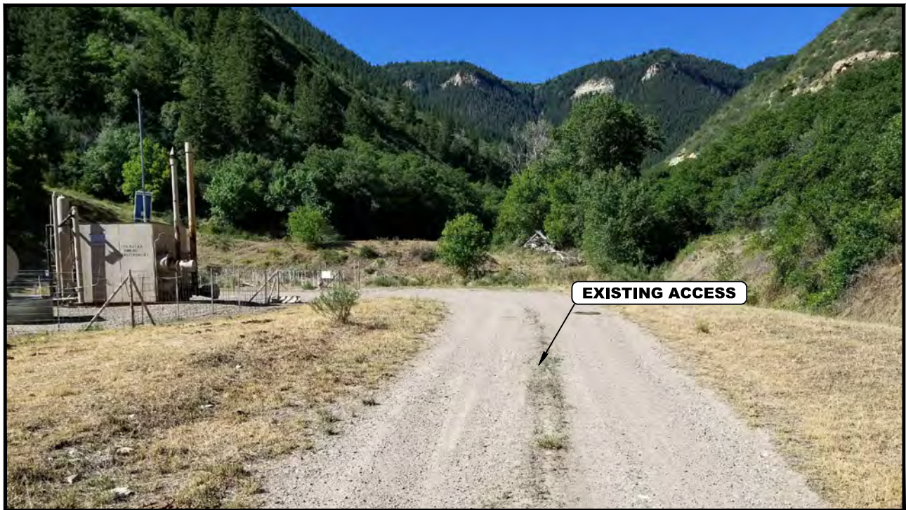
PHOTO: VIEW FROM BEGINNING OF EXISTING ACCESS
