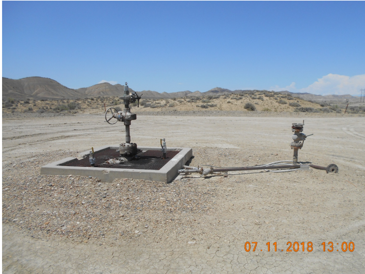
Injection Wellhead
