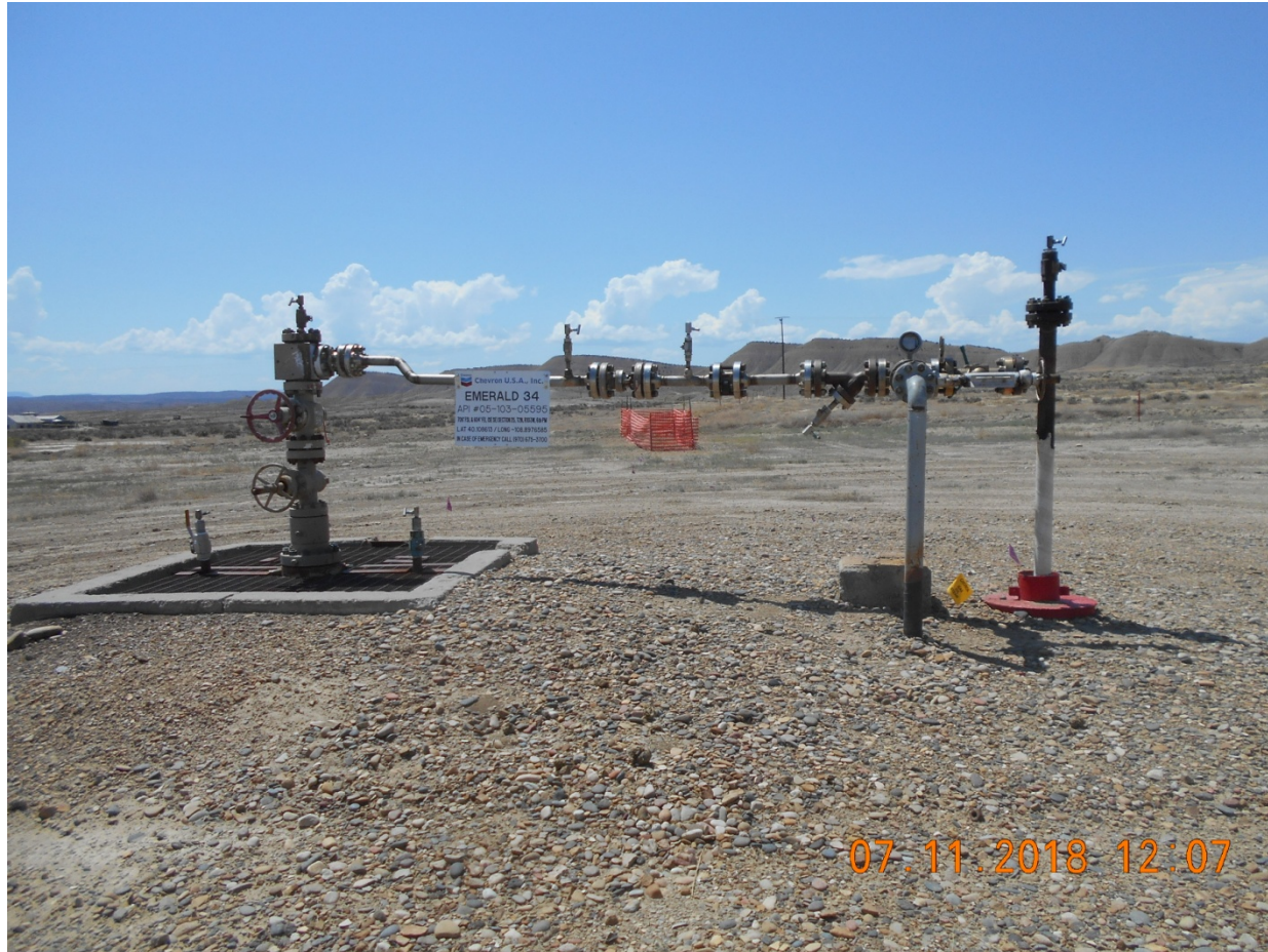
Injection Wellhead
