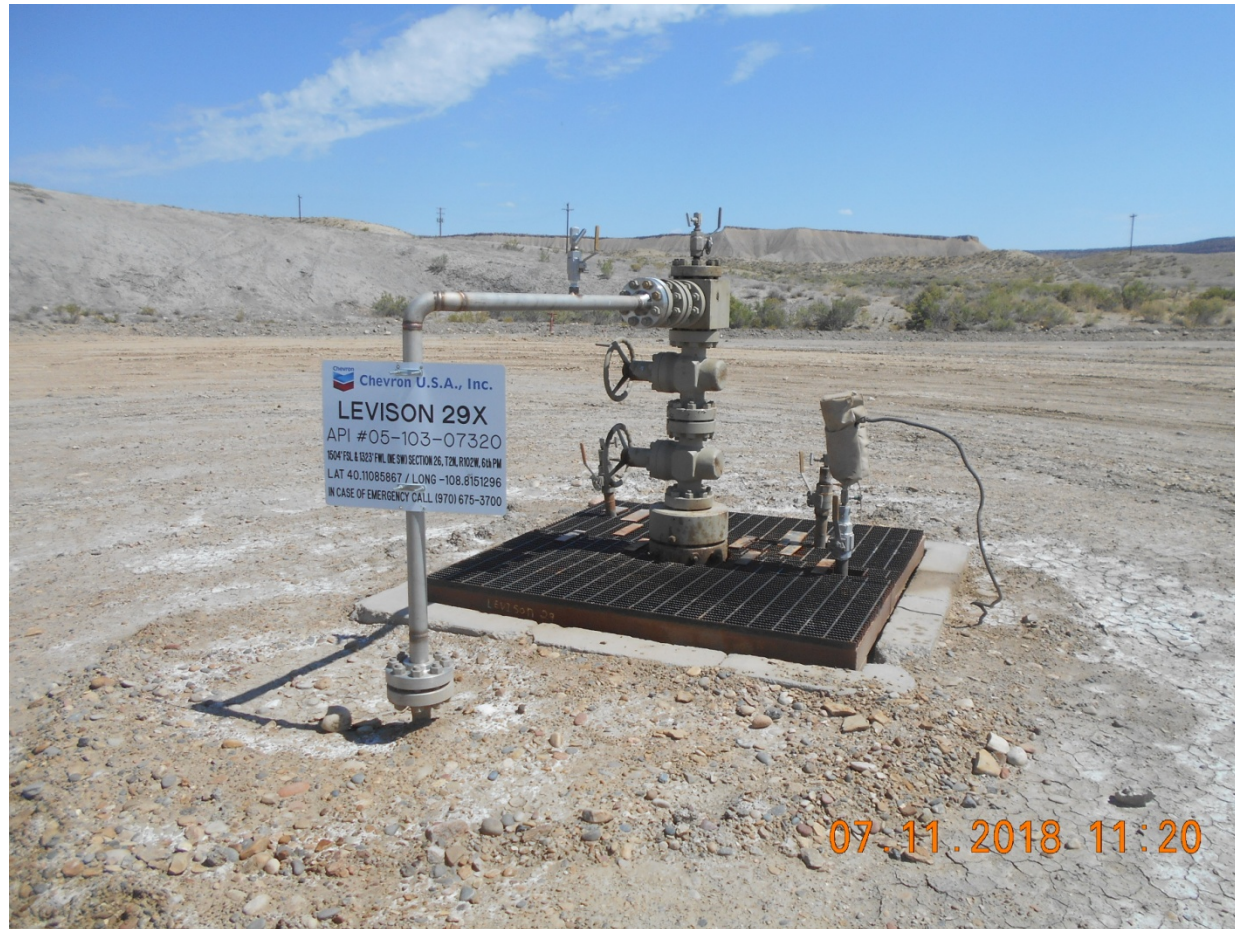
Injection Wellhead
