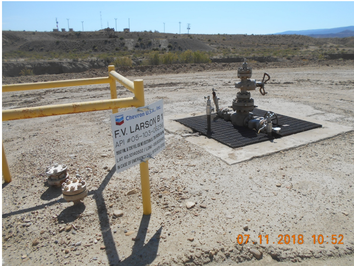
Injection Wellhead
