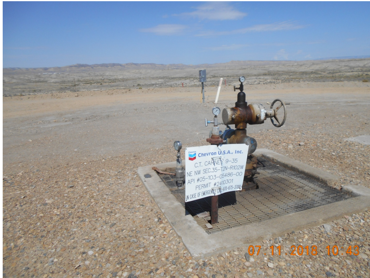
Injection Wellhead
