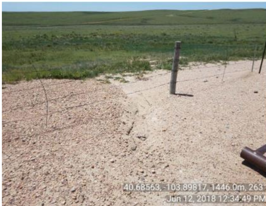
COGCC Photo 3: Stormwater erosion at S of wellhead
