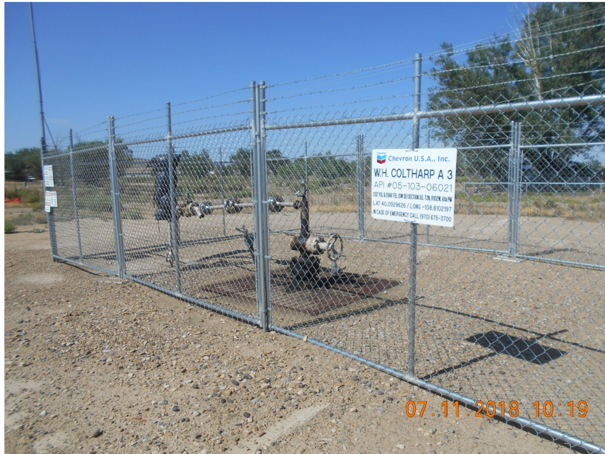
Injection Wellhead
