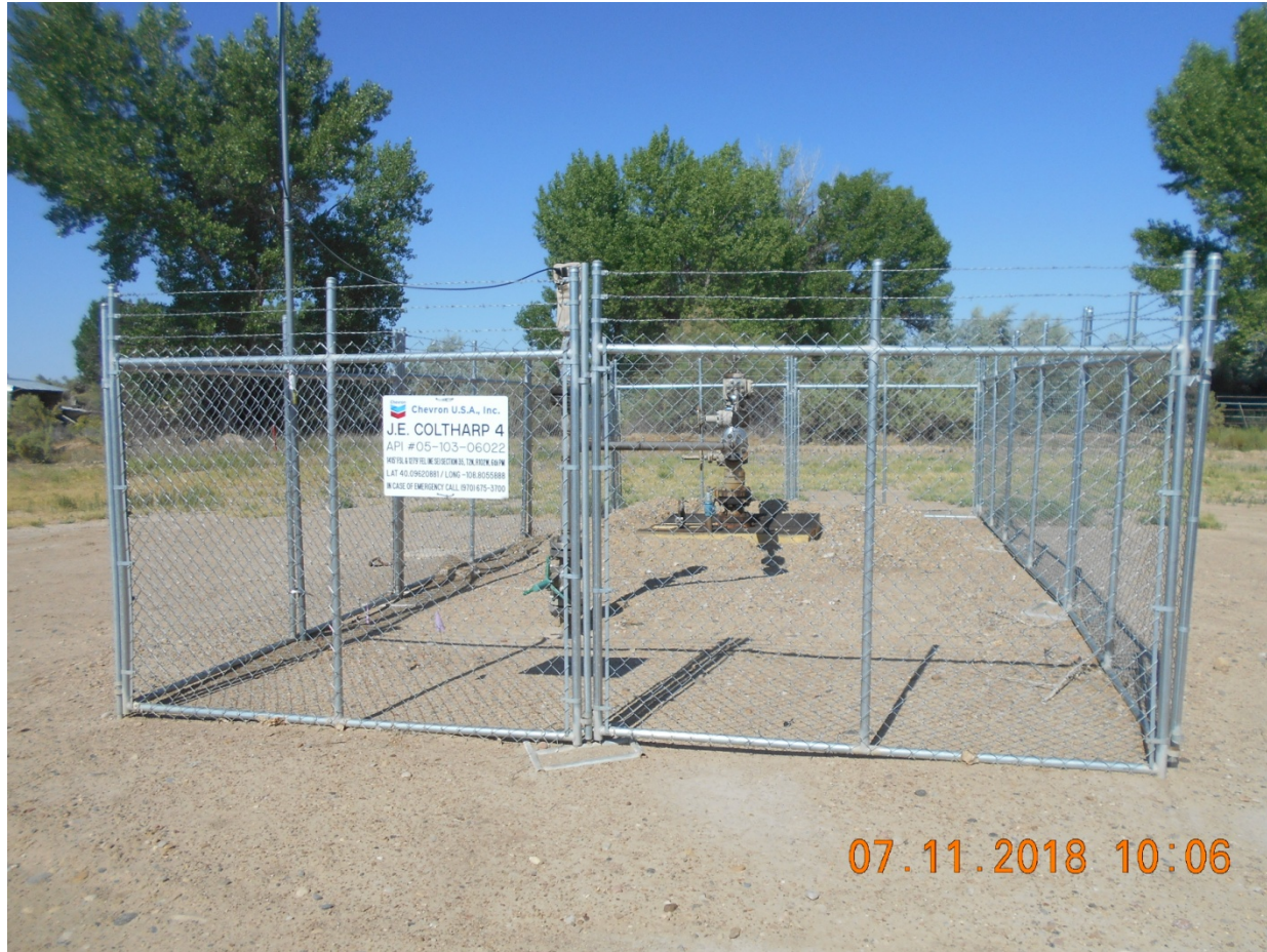
Injection Wellhead
