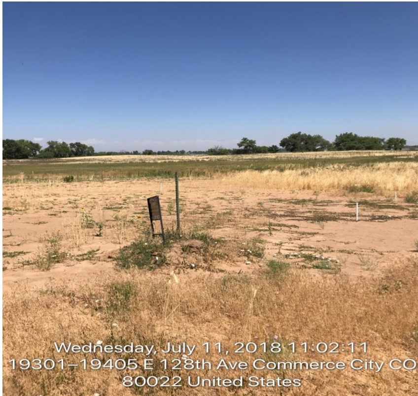
Photo#1P&Ad Battery Location
