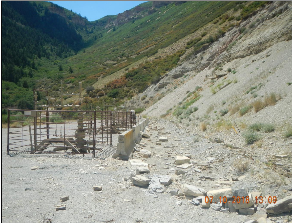
Fallen rock from unstable cut slope.
