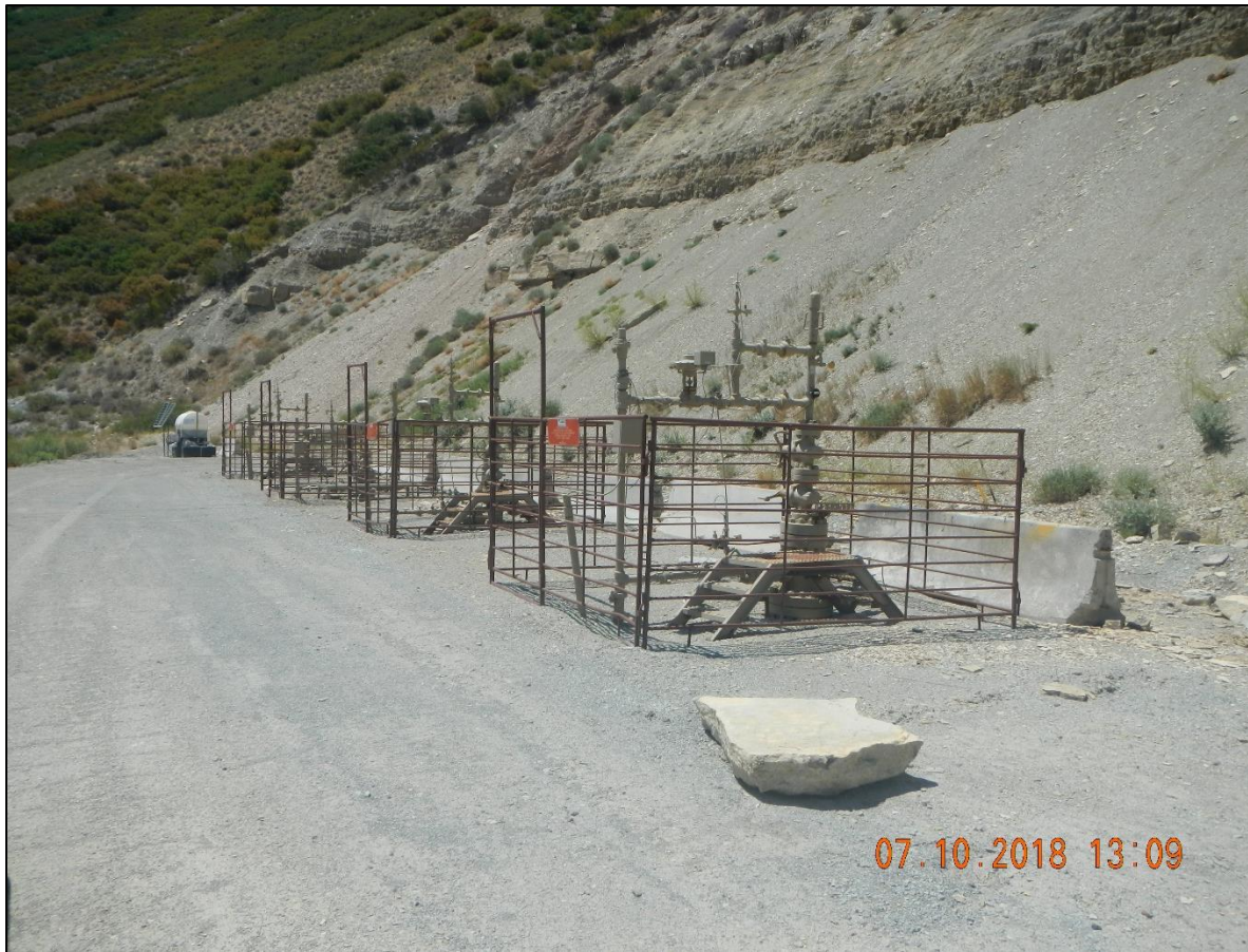
Fallen rock from unstable cut slope.
