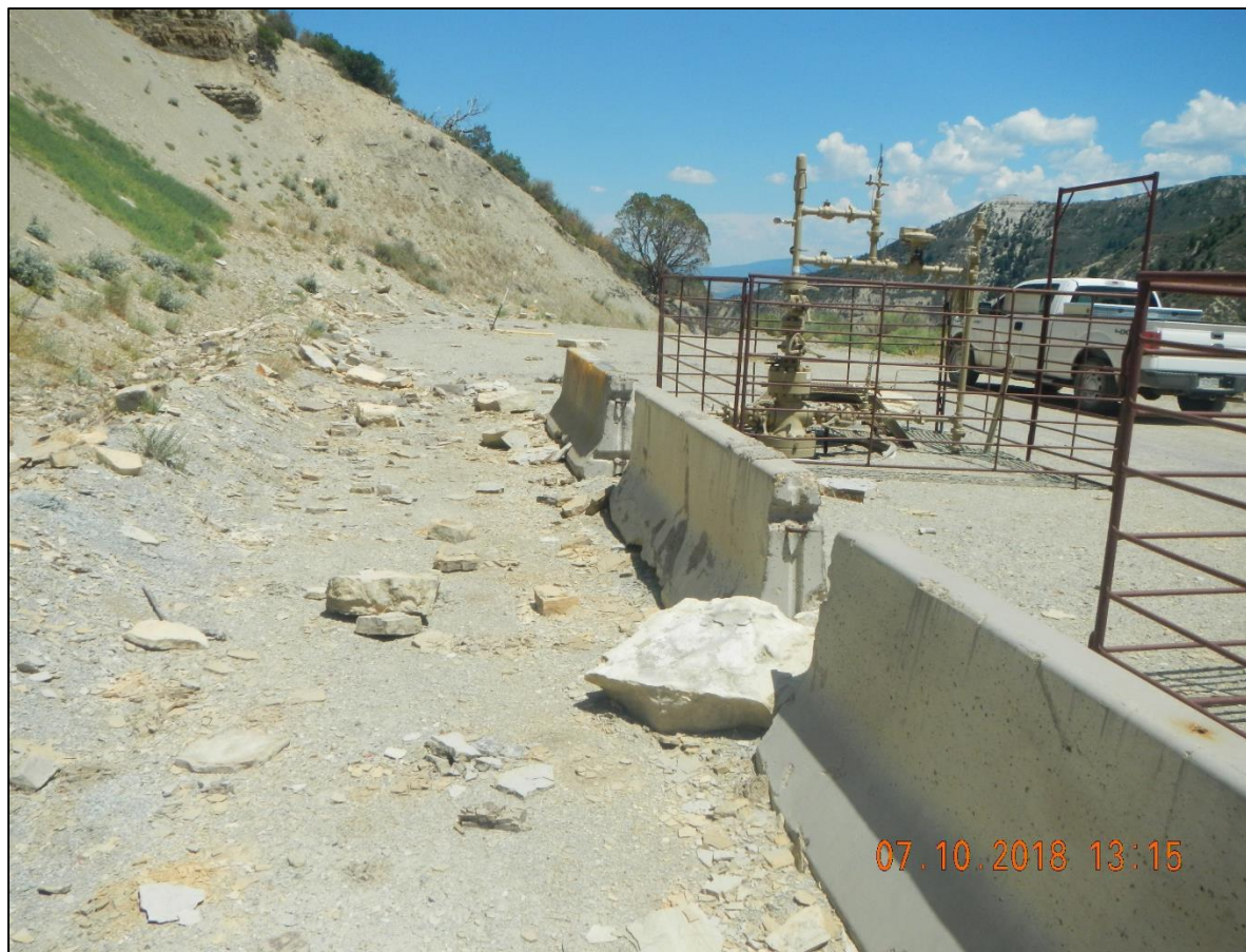
Fallen rock from unstable cut slope.
