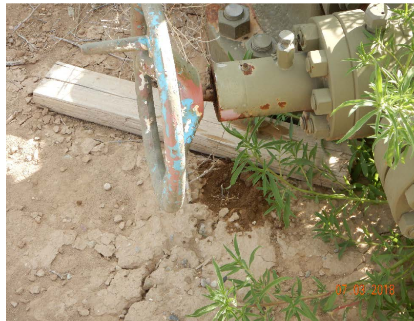
Photo #2 – Localized accumulation of oil-stained soil at wellhead.
