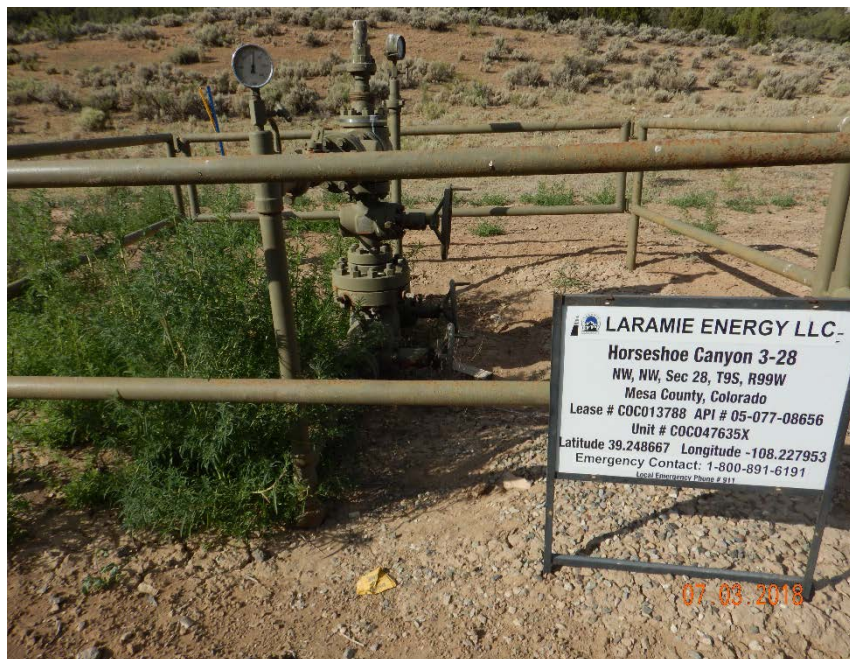
Photo #1 – Uncontrolled weeds at wellhead.
