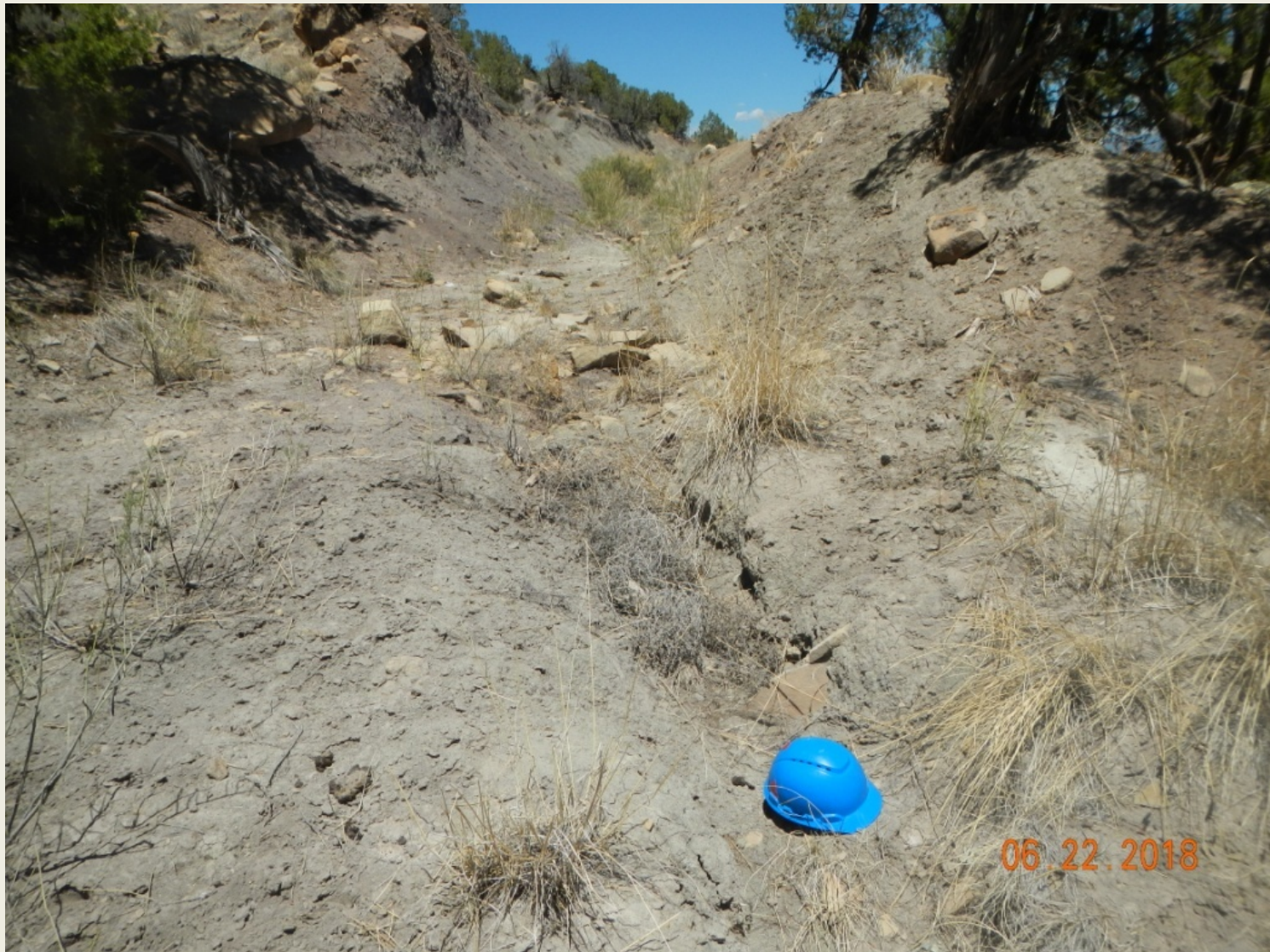
Photo 4. View of area in the southwestern corner of the project area where diversion feeds into an ephemeral drainage. Erosional channel approximately 2 feet wide and 18 inches deep is forming in this area.
