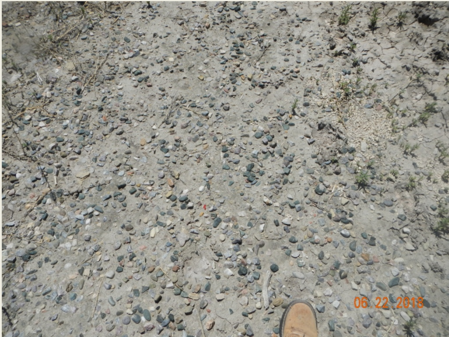
Photo 11. Birdseye view of gravel still in place in portions of the flat well pad surface.
