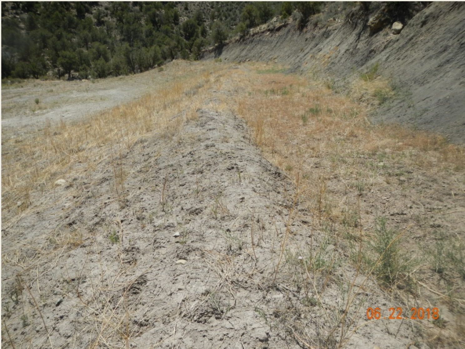
Photo 2. View of the western portion of the project area from the northwestern corner facing southward. Stormwater diversion is still in place and is full of sediment.
