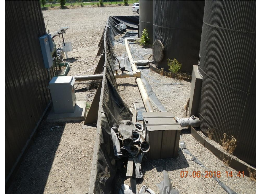
Penetration through liner and secondary containment ring where release reportedly occurred.
