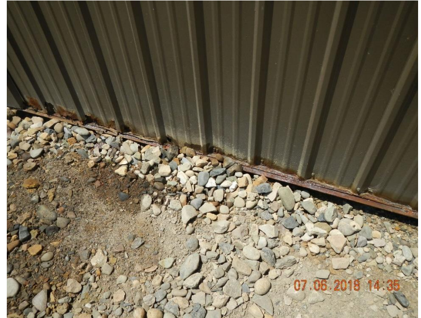
Southwest corner of injection pump house with wet/stained soil and corroded metal .
