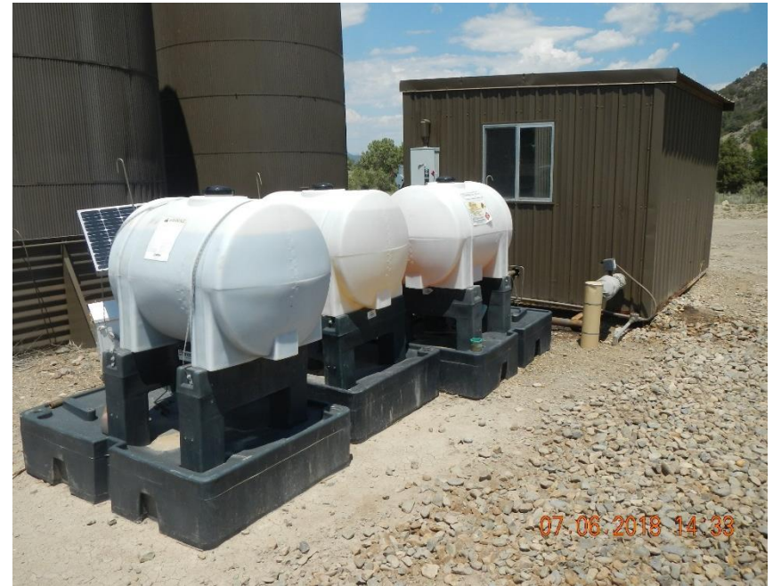
Chemical injection systems on secondary containment.
