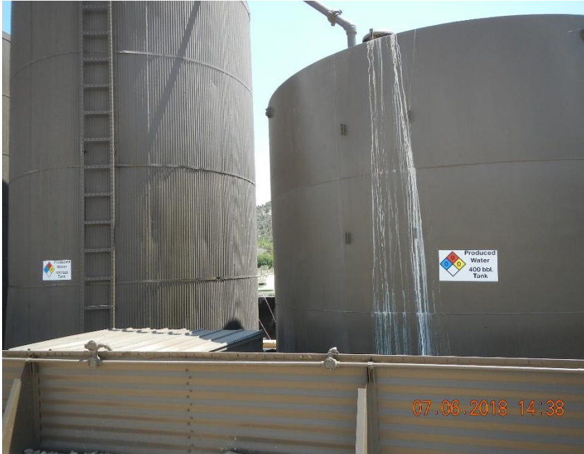
Staining on western produced water AST.
