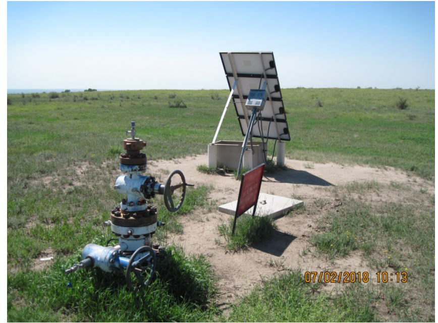
2. Wellhead equipment
