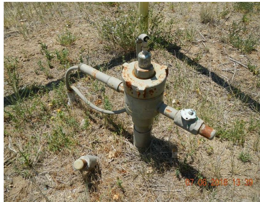
Fossett Gulch MW 34-5-14 #1 well head.
