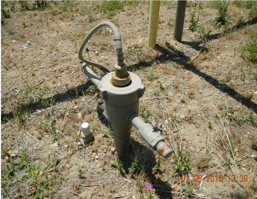
Fossett Gulch MW 34-5-14 #2 well head.
