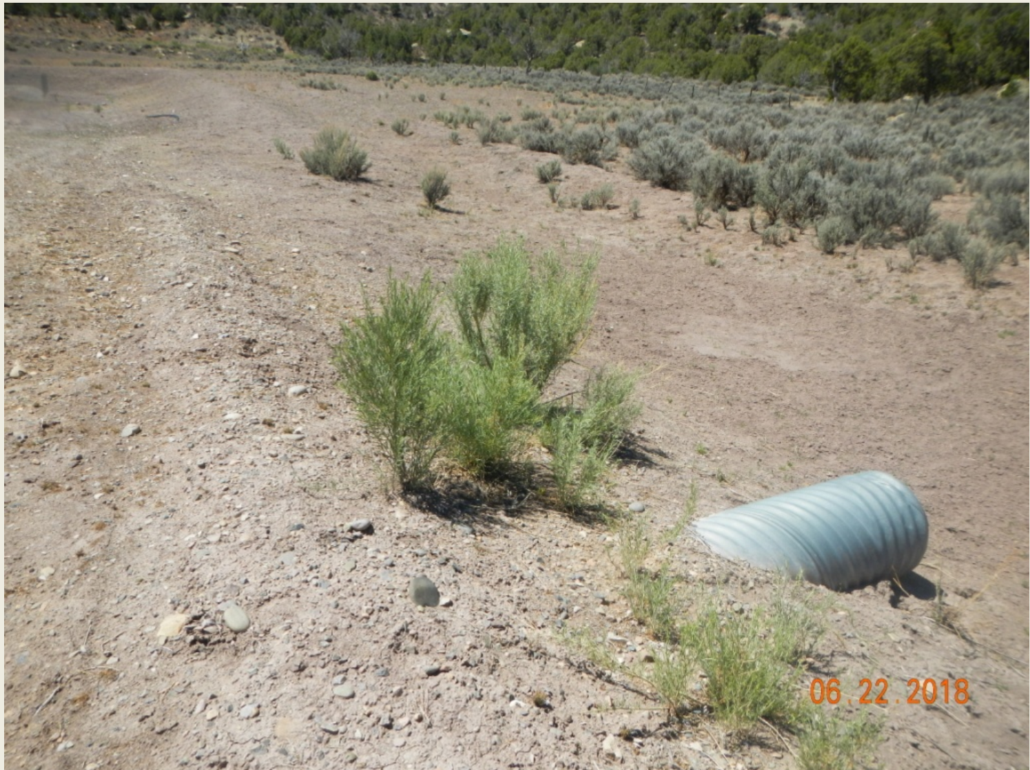
Photo 8. View of silt trap in the northwestern project area.
