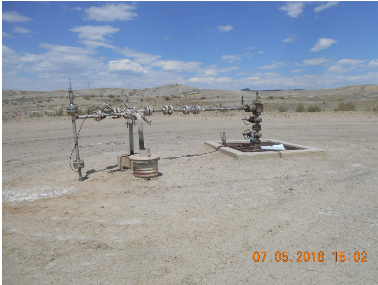
Injection Wellhead
